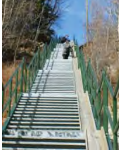
Staircases built with ramp for bicycles
