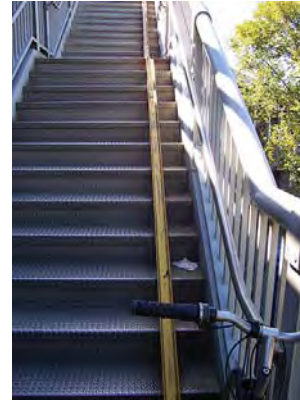
Staircases retrofitted with wheel gutter feature
