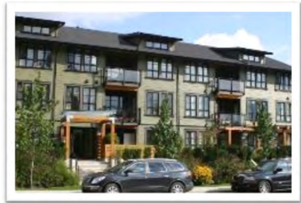
Example of Multi-Family Residential Development
