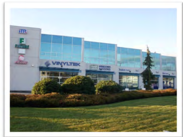
Example of Permeable Surfaces that support Stormwater Management
