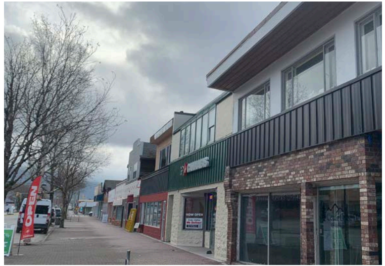
Above: In 2023, through a contractor, the City of Terrace removed the dilapidated canopy (shown at left) from the 4600 block of Lakelse Avenue. Businesses continued to work on facade improvements (shown at right) into 2024. More information is also available in the Development Services section of this report.
